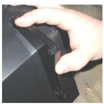
Step 8: <u>Bracket Installation:</u> Attach the "L" brackets to the back of the Square Plates on the Motor mounts, as shown below. Center the "L" bracket on the back of the Square Plate and mark the hole locations. Use a 3/32" drill bit for pilot holes. Install the "L" bracket flush with the top edge of the square plate. Secure the "L" brackets with #2 screws.
